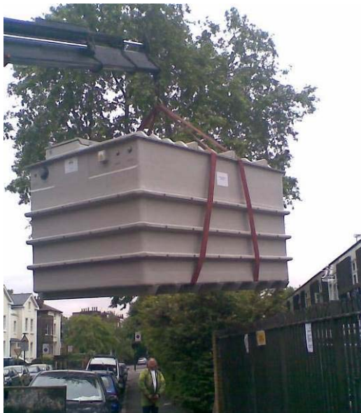
Fig 1a & 1b. Example Offloading from Lorry without steel support skid (strapped) and with steel support skid (fork lifted).
