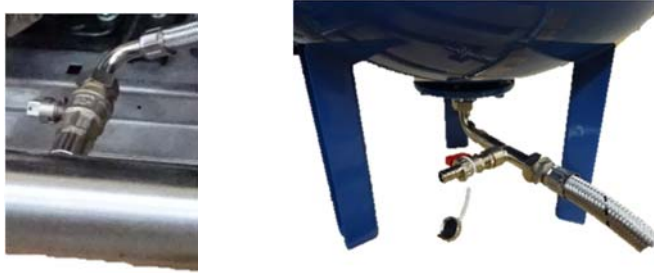
Fig. 1.5a & b Isolation valve on pipework & Flexible hose with drain cock on vessel (non-flow through vessel shown)
