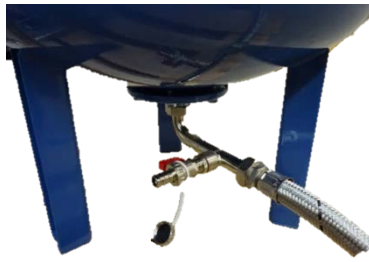
Fig. 1.5a & b Isolation valve on pipework & Flexible hose with drain cock on vessel (non-flow through vessel shown)
